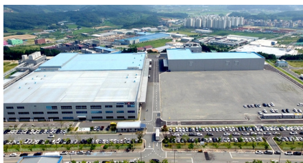
Fig. 3 Fuel Cell Manufacturing Plant
